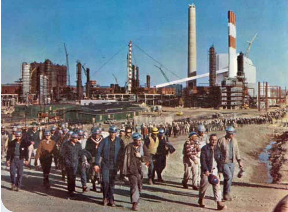
Suncor workers leave the oil sands plant, circa 1967.
